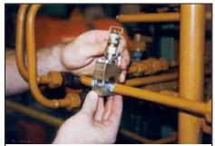
•Clamp the valve mount to the pipe
