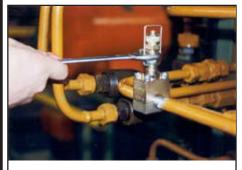
•Using an open jawed wrench (without extension), screw in head joint in clockwise direction as far as it will go.
